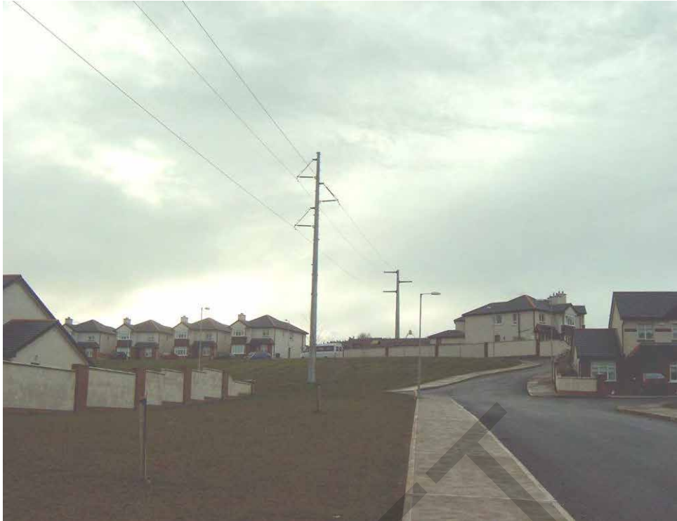
Figure 4.14: 110 kV Monopole Overhead Line in Cork
