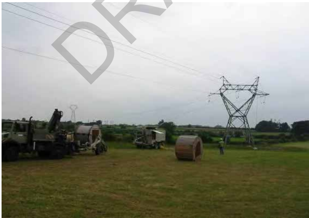
Figure 7.14: Typical Stringing Equipment
