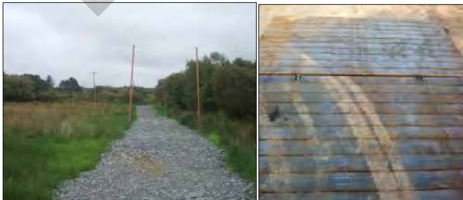
Figure 7.4: Temporary Stone Road and Wooden Sleepers
