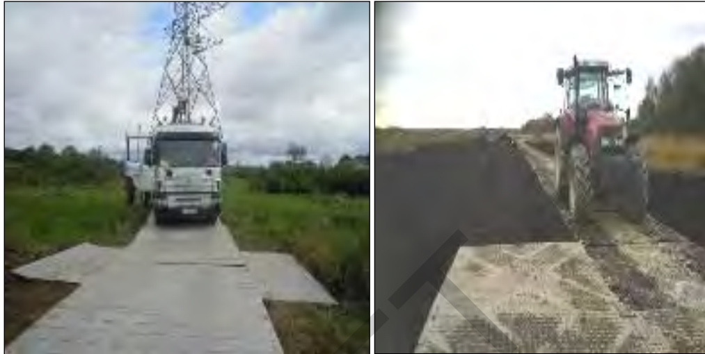
Figure 7.3: Temporary Aluminium and Rubber Panel Tracks
